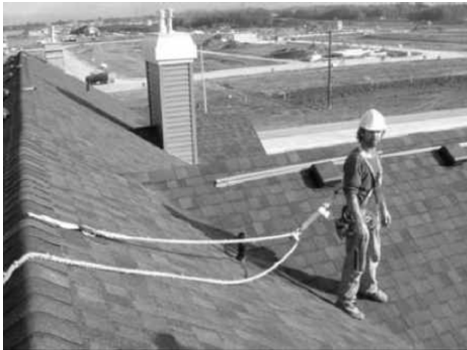
Figure 10.5 Another example of a Fall Arrest System
